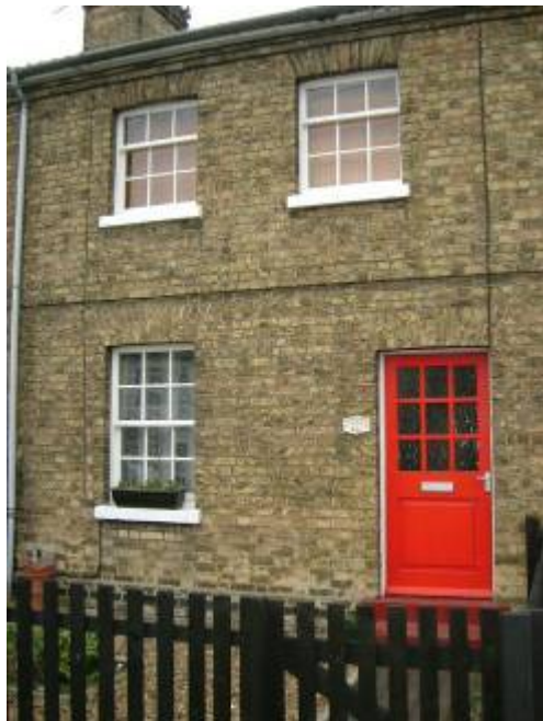
Typical cottage: Southern terrace
