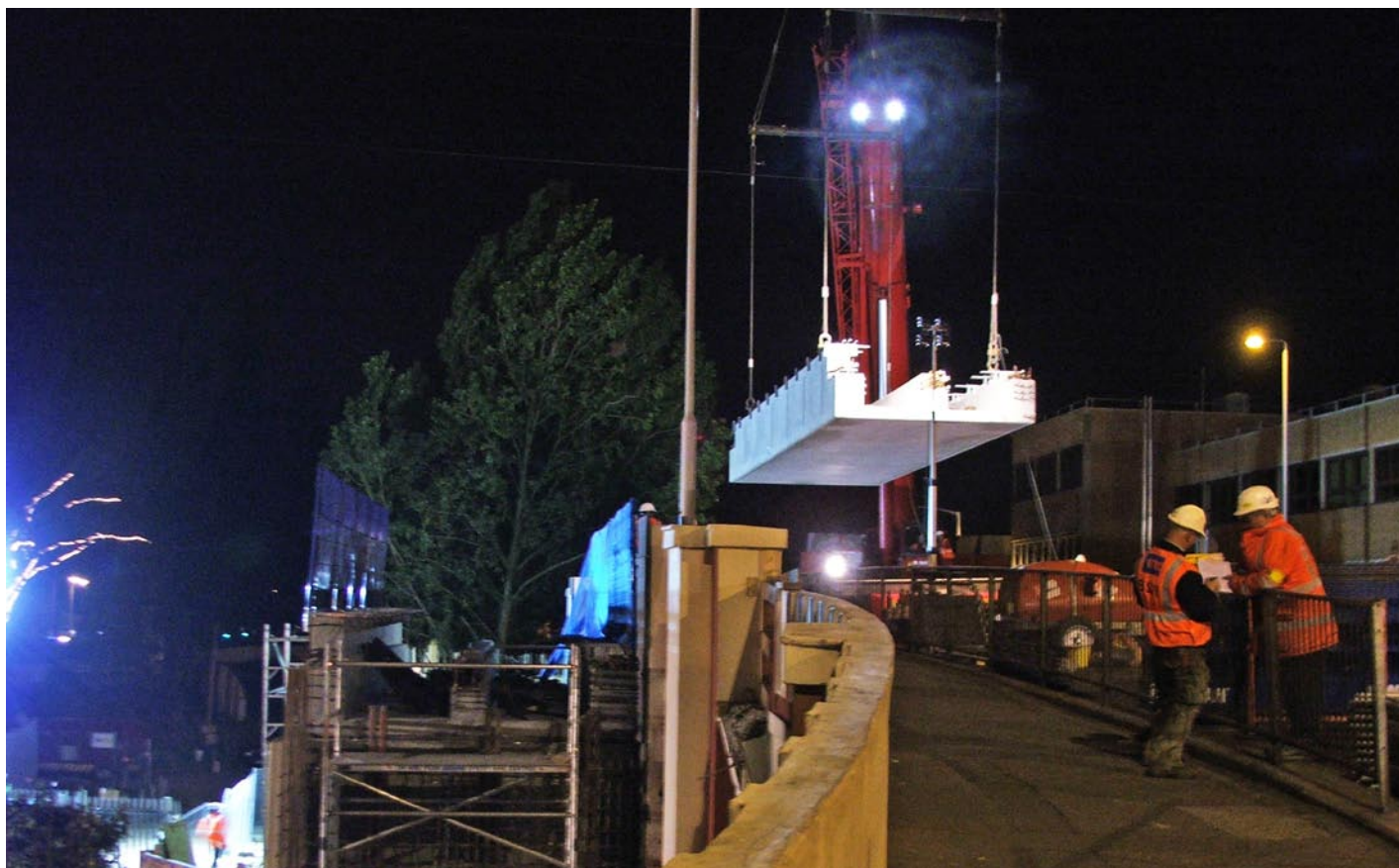
Town Rail Bridge Structural Repairs
