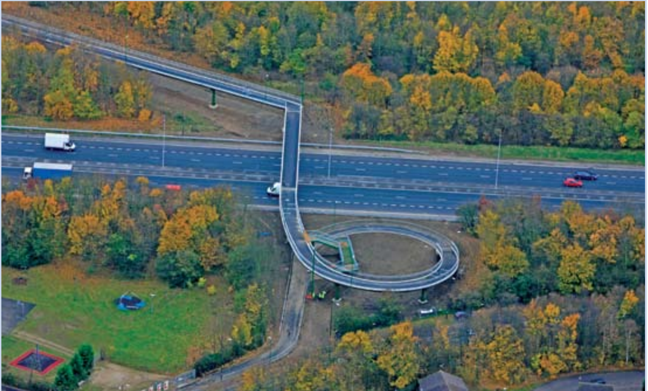
Fletton Footbridge, located between Junctions 2 and 3
