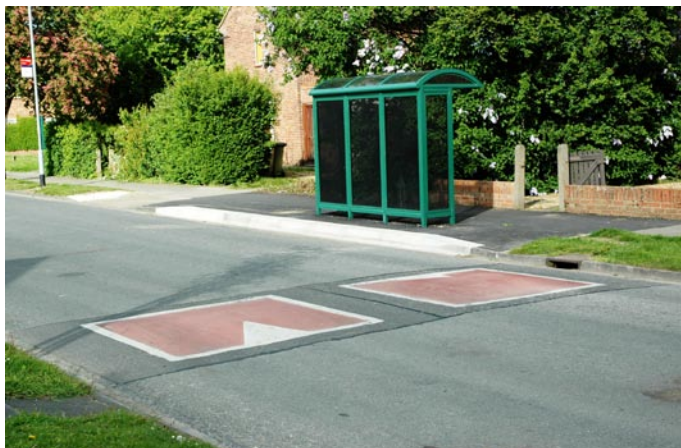
Eastfield Local Safety Scheme
