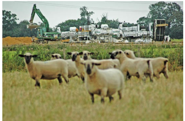
Work on the Thorney Bypass
