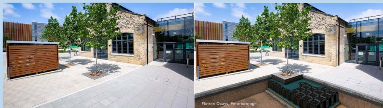
Figure 3-4: Wildlife areas, rain gardens and tree pits were incorporated into Fletton Quays redevelopment (photo provided by GreenBlue Urban)
