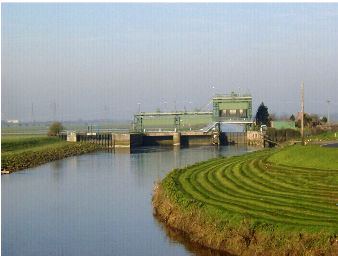
Figure 5-3: Dog in the Doublet sluice when the tide is not so high. Source: Environment Agency.
