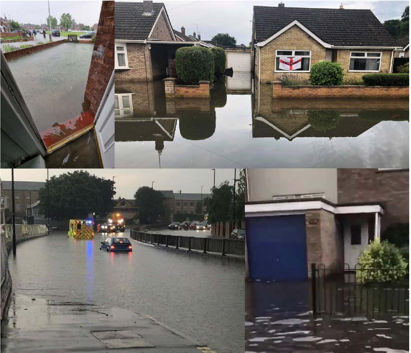
Figure 7-5 Flood events in July 2021
